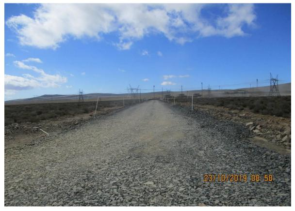
Photo: Layer works on permanent access road.
