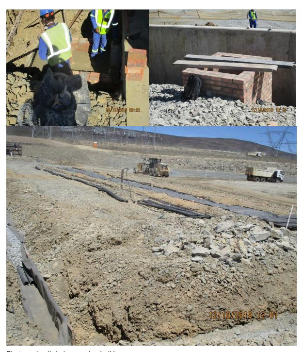
Photo: subsoil drainage mine hall in progress.
