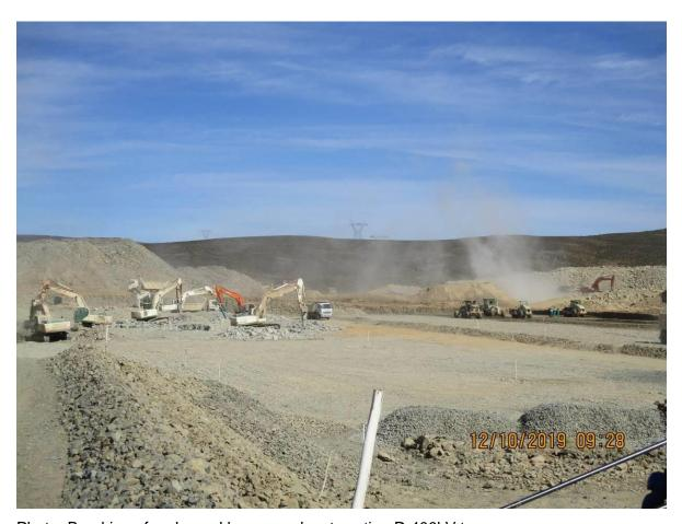
Photo: Breaking of rocks and layers works at section D 400kV terrace.
